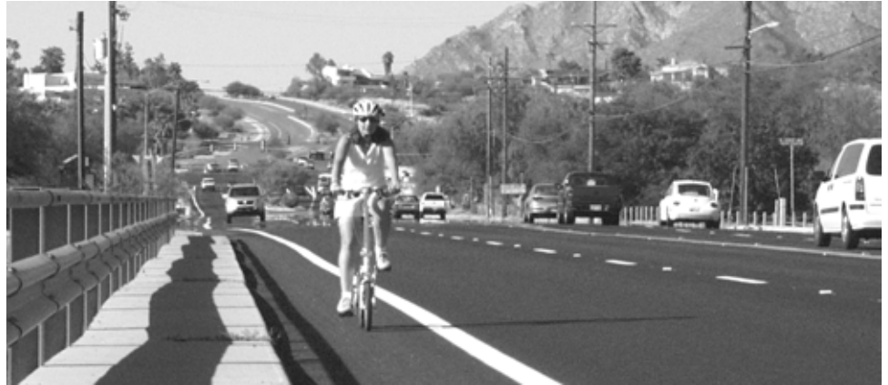
25 miles of new bike lanes and sidewalks will be constructed during this year. Shown here is a new bike lane over the Rillito River at 1st Avenue.
